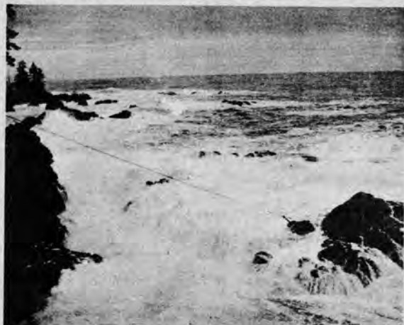
A stormy day off Pachena Point. Cable runs from flat rocks to top of 150 foot cliff. Freight was winched up cable by small gas engine. Calm weather required.
